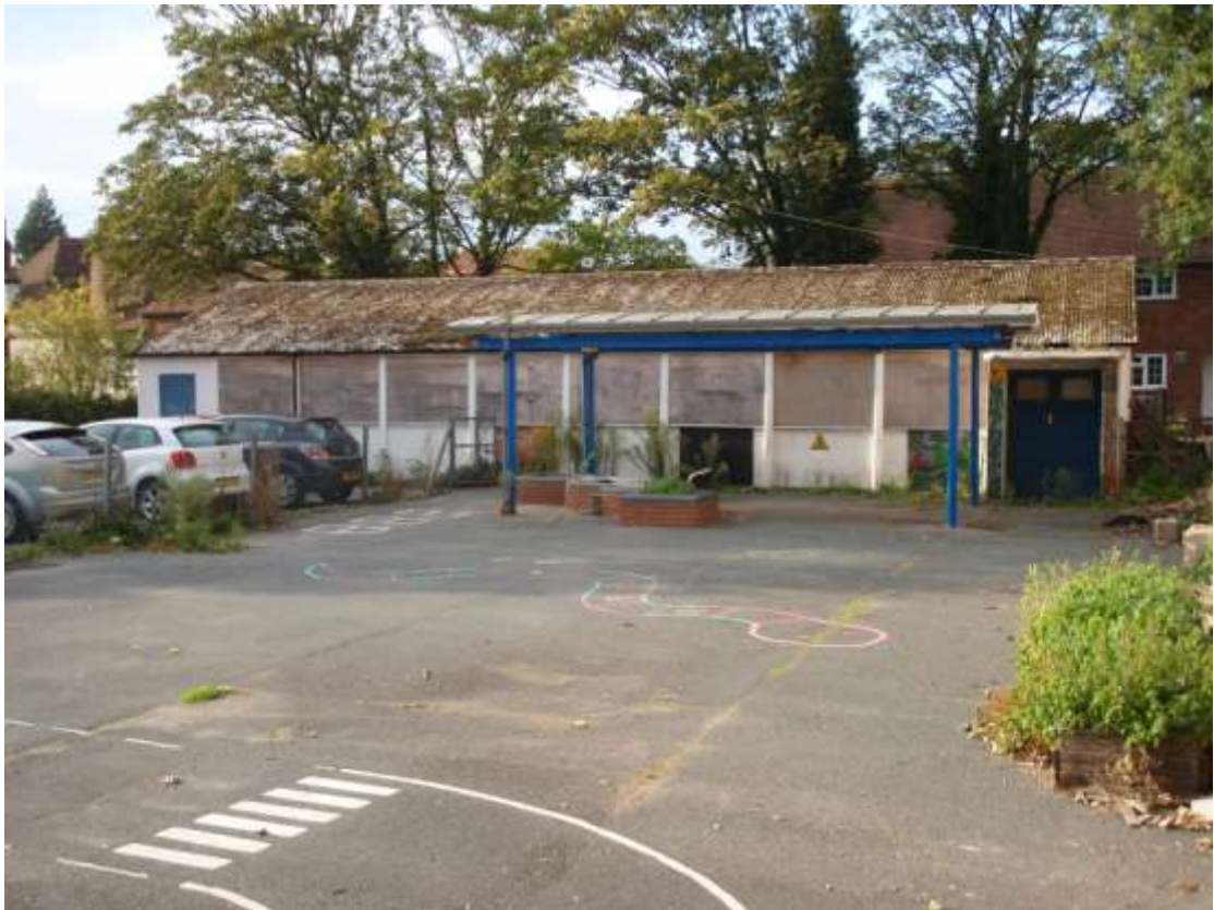
Plate 6. Viewing the Site (looking north)
